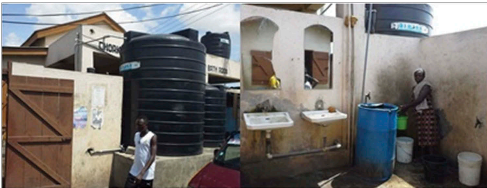
Figure 3. Left: Chorkor toilet and bath facilities; right: pipe-water system. Source: Field Survey, 2014.
