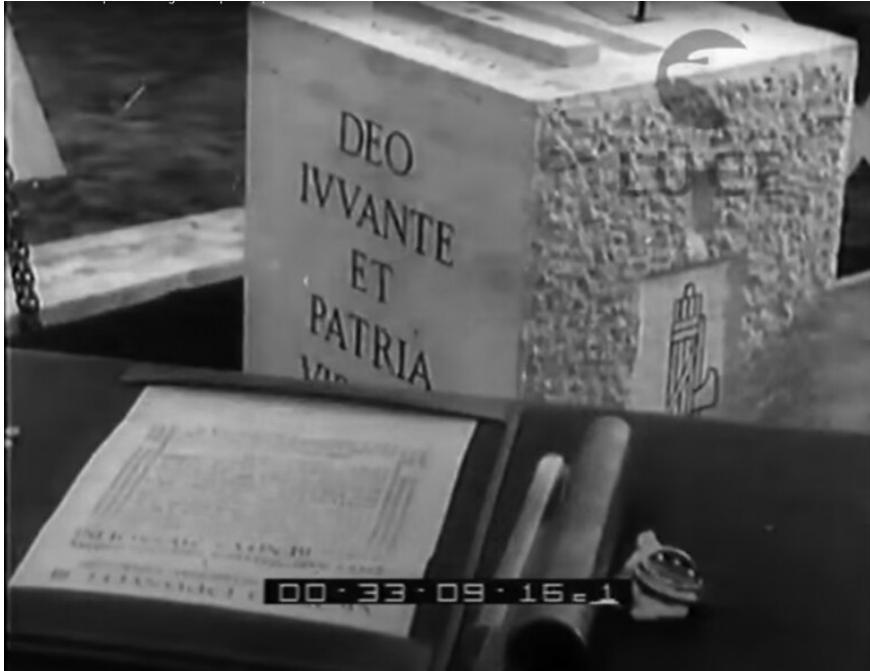
FIGURE 8 Video still from Giornale Luce , B1188, October 27, 1937, showing the contents of the foundation deposit for the office blocks at the site of the world exhibition (00:33:09)
