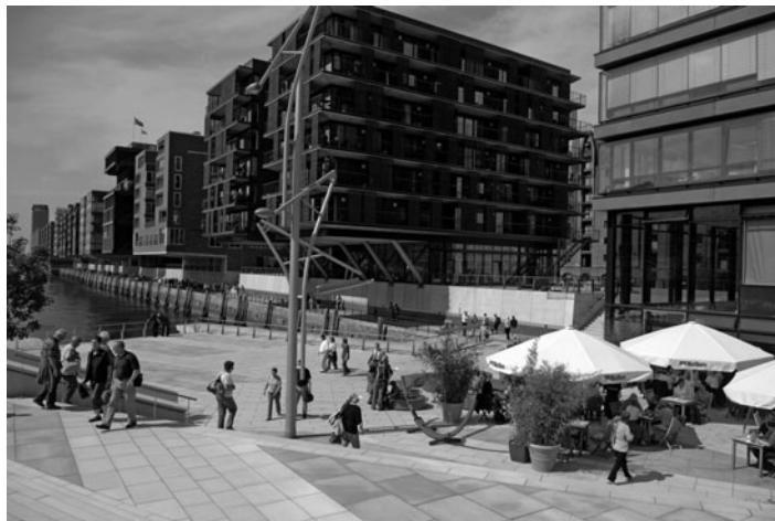
Figure 4. Basements of buildings, usual situation. Source: ELBE&FLUT/Thomas Hampel.
