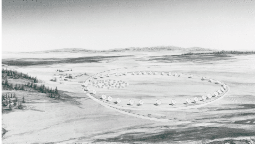
FIGURE 1.2. An artist's impression of the millimeter array (MMA). Current plans involve a joint US European effort to build up to 64 antenna's each focusing the signal onto about 6 detectors with 2 polarizations, meaning that a total of 640 superconducting detectors will operate simultaneously.
