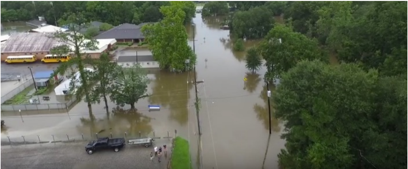
Figure 4: Downtown Springfield and parts of Highway 22 towards Ponchatoula captured by Dev/Null, “Louisiana Flood 2016—Springfield Hwy 22—Drone Aerial Footage.”
