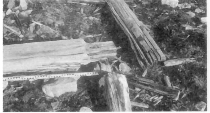
FIG. 7. The SE corner of het Behouden Huys with the southern beam carved out so that it fitted over the squared eastern beam (photo by L. Hacquebord).
